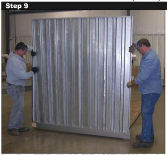
Install a SIDE WALL SUBASSEMBLY by inserting a side edge into one of the lock strips.
