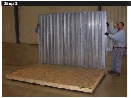
Position BACK WALL SUBASSEMBLY as shown above. NOTE: Install on one of the lengthwise sides of the FLOOR BASE.
