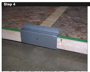
Install a FLOOR SEAM COVER PLATE on both sides to the center of the two joined wooden floors with a ½" x 2" lag screw (part no. 22061) – one bolt per face joint on each side for the wooden floors.
