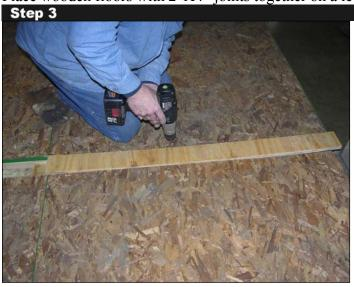
Using 20pc of 2" long wood screws fasten the plywood spacer strips directly to the 2"X4" joints. Evenly space wood screws along entire length of spacer strip. NOTE: Attach screws evenly to both 2x4's.
