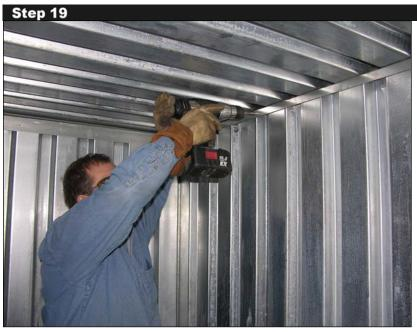
Secure roof to front and back walls with 16pc
