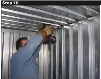
Fasten the ROOF to the front and back walls with 8pc of 1" long self-tapping screws (part no. 31806; 4 pcs. per wall). There are no predrilled holes. Space screws evenly across both walls.
