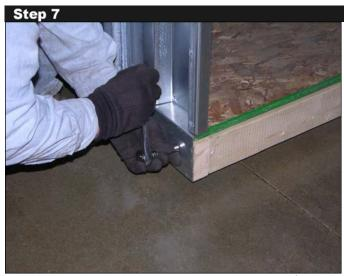
Secure BACK WALL SUBASSEMBLY to the wooden floor installing ½"x 2" lag screws into the 5 predrilled holes in the bottom flange. The BACK WALL will fall over until it is attached to at least one SIDE WALL SUBASSEMBLY. Support the back wall until it is attached to at least one side wall and *both* walls are securely lagged to the wooden floor.
