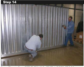
Install another SIDE WALL SUBASSEMBLY on each side. Then install 10pc ¼"x2" lag bolts to secure walls to wooden floor. There are 5 predrilled holes at the bottom of each SIDE WALL SUBASSEMBLY.
