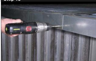
Fasten the ROOF SEAM COVER PLATE to roof and walls with 4 self-tapping screws. (2 screws at each end of the cover plate)
