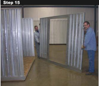
Photo shows FRONT WALL ASSEMBLY of STOR-912 without door.
