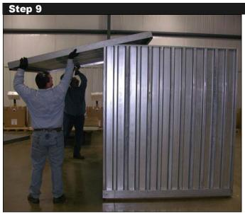
Place the ROOF WALL SUBASSEMBLY on top of the wall panels. The perimeter flange of the ROOF WALL SUBASSEMBLY must be on the outside of the wall panels. Pull/tap the ROOF WALL down until it seats onto the tops of the supporting wall panels.
