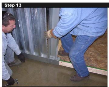
Insert the flange of one side of the SIDE WALL CONNECTOR into LOCK STRIP. Then, apply a LOCK STRIP to other flange of the SIDE WALL CONNECTOR. Repeat this step with the opposite side wall.
