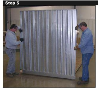
Insert the edge of one SIDE WALL into one of the LOCK STRIPS installed in Step 4.
