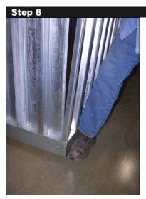
Insert a side edge of the remaining SIDE WALL into the other LOCK STRIP. Brace the bottom of the SIDE WALL while inserting the edge.
