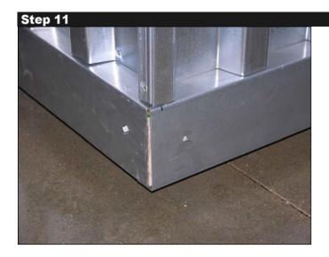
Secure both side walls to the wooden floor using ½" X 2" lag bolts into the 5 predrilled holes on each side.
