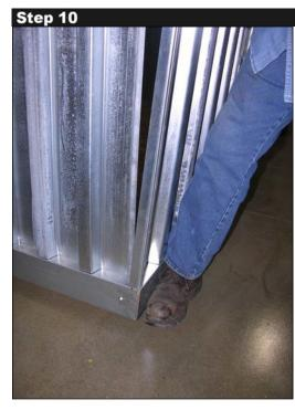
Install another SIDE WALL SUBASSEMBLY on opposite side of BACK WALL. Brace the bottom of the side wall while inserting it into LOCK STRIP.
