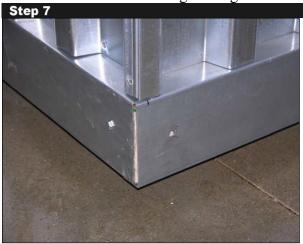
Fasten both SIDE WALLS to the wooden floor with ¼"x2" lag screws (22061) installed through the 5 predrilled holes in the bottom flange of each SIDE WALL.
