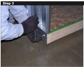
Fasten BACK WALL to the wooden floor by installing ½"x2" lag screws (part no. 22061) through the 5 predrilled holes in the bottom flange of the BACK WALL. Continue supporting the BACK WALL until is fastened to at least 1 SIDE WALL SUBASSEMBLY this is also lagged to the wooden floor.
