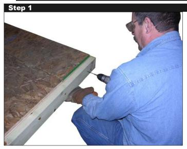
Fasten a 2"x 4" to one of the 9 foot (STOR-912) or 6ft. (STOR-612) sides of each WOOD FLOOR BASE. Attach 2x4's  $\frac{3}{4}$ " from top of floor bases (thickness of plywood) using 6pc - 3" long wood screws as evenly spaced as possible.
